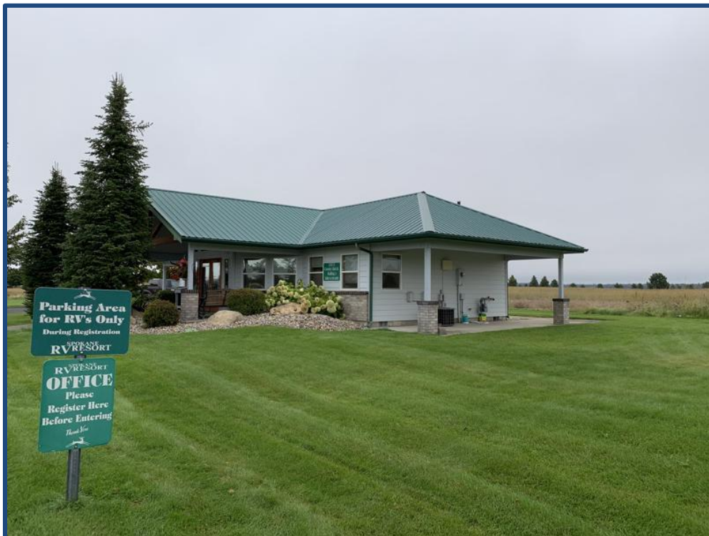
Office facing northeast
