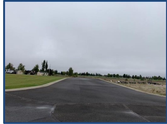
Typical common area road
